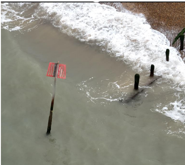
Image: Defected marker to be repaired
